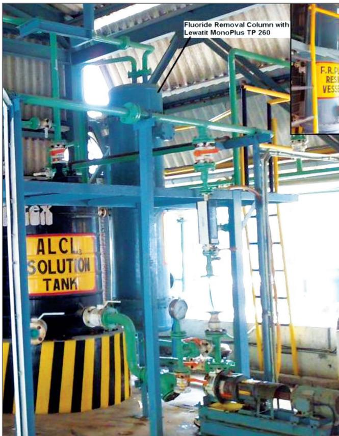
Figure 4: Fluoride Selective Ion Exchanger Operated At A Major Chemicals Manufacturing Company In Gujarat, India
